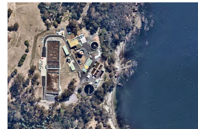
Image: Blackmans Bay Sewage Treatment Plant
